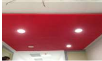
Suspended false ceiling in loading area
