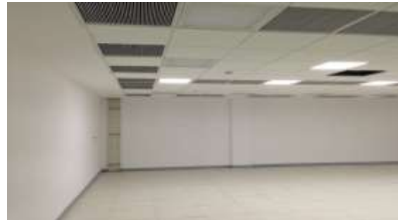
Main floor area with usage of Armstrong false ceiling, Metro Grid flooring , Promatec fire rated partitions & cable trays above and below false ceiling by legrand
