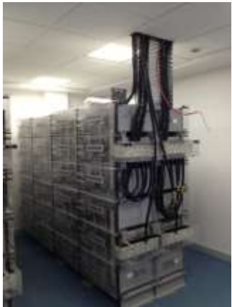
Completed battery bank
