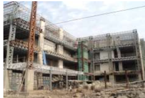
Truss installation of the data center
