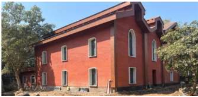
Views of the structure
