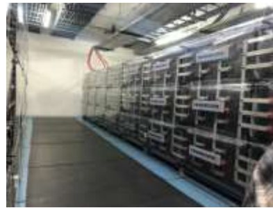
New Battery Room
