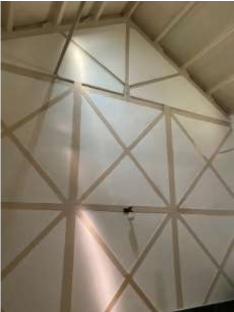
Internal work after highlighting the wooden bracing
