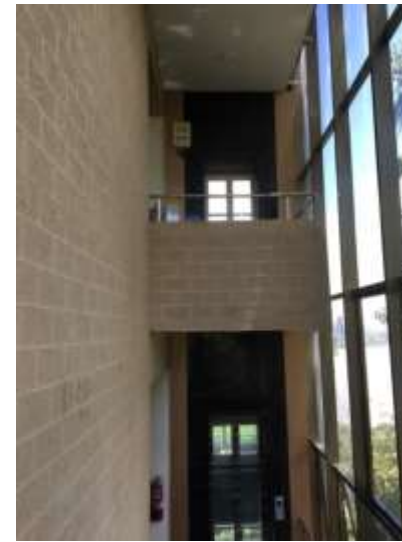
Use of Malad stone plaster in the interior
